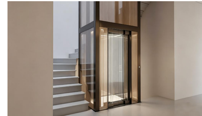
This Also Applies to Standard Elevators With Shafts.
