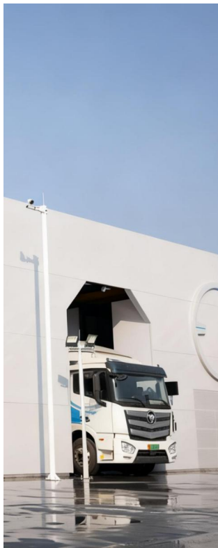
Battery Swap Station
